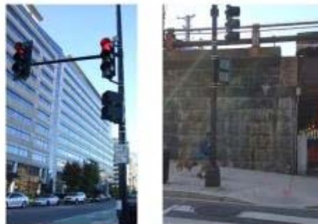
Left: The misaligned pedestrian signal head at 1 st street in the northeast quadrant. Right: The misaligned pedestrian signal head at 2 nd Street in the southwest quadrant.
